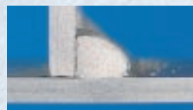
Without start-up program – fusion defects at beginning of seam
